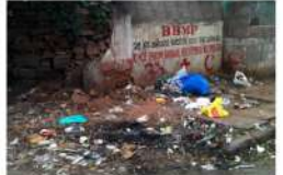
EXISTING ROAD CONDITION
