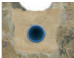
open trench installation in sandbed
