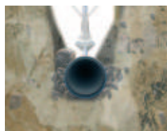
open trench installation without sandbed, ploughing and milling
