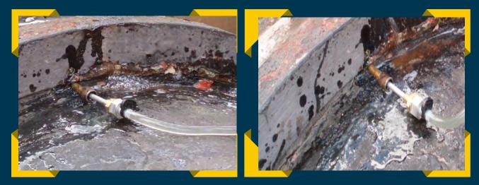
These images were taken at a live site repair carried out at Tottenham Holder Station on a 38" lead yarn main. In the second image, Ecoseal has been successfully injected. The lack of bubbles indicates the leak has been repaired.
