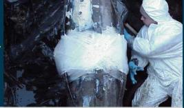
The USA Uitility company was struggling with a significant challenge related to a 4" High Pressure Clamp. This issue has arisen due to the deterioration and corrosion of the gasket, a vital component within the clamp system. The consequence of this gasket corrosion is the occurrence of unwanted and
