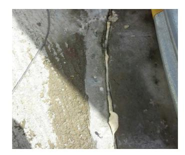
The process of Resin Injection was used to repair cracks in the bunded area of the treatment plant, where water was percolating through construction joints as shown in this image.
