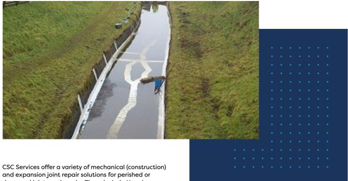
CSC Services offer a variety of mechanical (construction) and expansion joint repair solutions for perished or damaged joints and cracks. These include Hypalon bandage systems which are secured and sealed to each side of the expansion joint or crack using epoxy resin adhesives. DWI approved products are available. These systems are chemical resistant and will alleviate water egress and ingress whilst allowing the expansion joint to accommodate movement.
