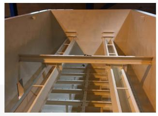
These multi-media steel filter tanks are extremely expensive to replace and if they need to be, can cause significant disruption to operational services due to decommissioning, removal and construction of new steel tank filters. Tank refurbishment offers a cheaper and quicker alternative and can allow remaining filers and operations at a treatment plant to continue.
