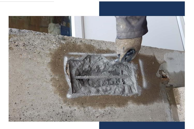
The age of the buildings combined with environmental factors has resulted in spalling of concrete at various areas across the hospital. Defective concrete was removed and concrete repairs undertaken using cementitious repair materials.
