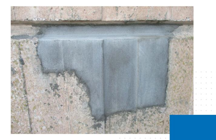
Over ten tonne of specialist repair mortars and structural strengthening products were used to rectify the degradation of reinforced concrete at various areas across the station.
