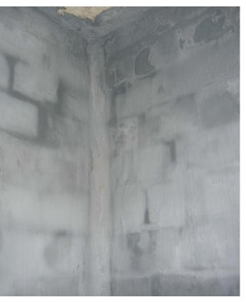
The chamber forms part of the surface water drainage system and is also the authorised minor discharge route for waste condensate water being discharged from the power station. Although the chamber was intact, there were voids in the mortar and cracking around pipe penetrations. The defects needed to be repaired to ensure environmental compliance is maintained. A protective lining was required that would tolerate the heat from the water being discharged.
