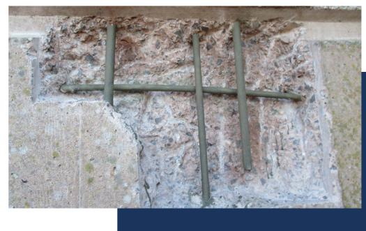
A combination of environmental exposure, water ingress and the age of the station building, had caused spalling in areas, including the flask bay and turbine hall.
