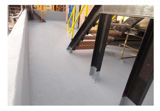
CSC Services installed a Sika Liquid Plastic Roof to a Pumphouse Flat roof at Hartlepool Power Station for EDF Energy. Sika Decothane Ultra was specified for this system, which was inclusive of Reemat and Decotrim Type F. The roof was approximately 205 square metres.
