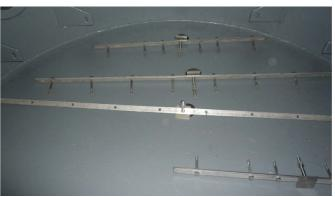
Following the removal of lateral supports and internal pipework, chemical resistant lining Ceilcote 242 Flakeline by International Paints was used for the vessel refurbishment. Ceilcote 242 Flakeline is a flake filled vinyl ester coating with excellent resistance to organic and inorganic acid solutions and many aliphatic solvents. It has a designed lifetime of ten years. The coating system comprised of primer and four coats roller applied.
