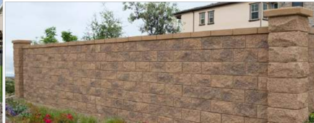
TUSCANY VARIEGATED BLEND 6x8x16 CMU-SPLIT FACE BLOCK-WITH STONEGATE COLOR MORTAR, 8x2x16 WHEAT CAP, PILASTERS BY GRACO BLOCK
