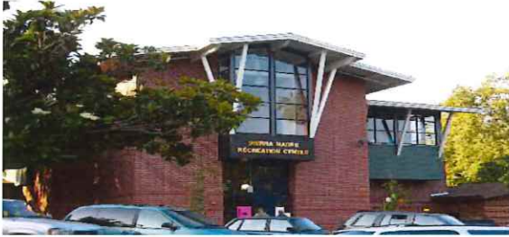
Sierra Madre Youth Activity-Teen Center New 1st Floor Entry & 2nd Floor Addition City of Sierra Madre
