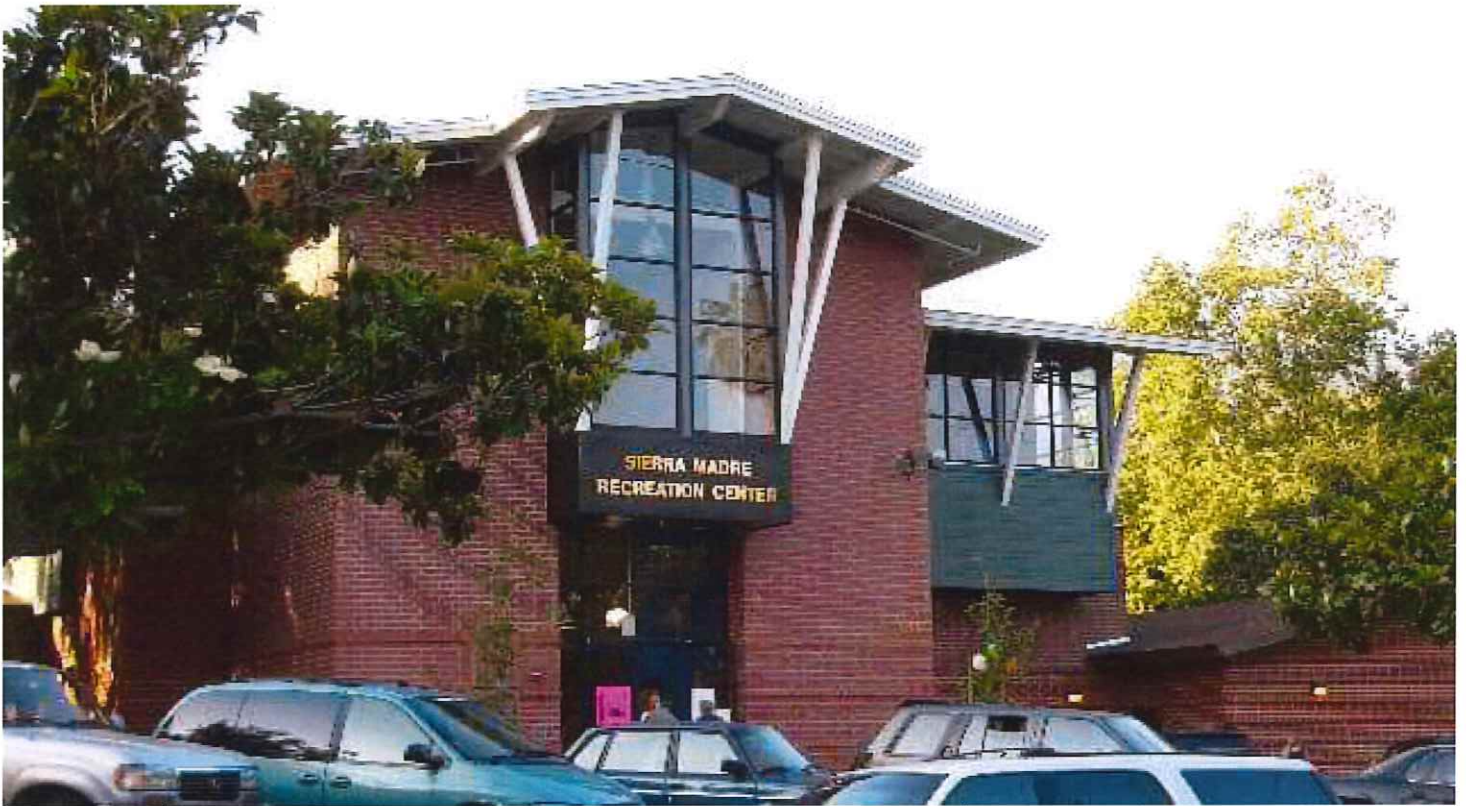
New 2 nd floor Teen Center with a "tree house" theme is built over existing 1 st floor Community Center
