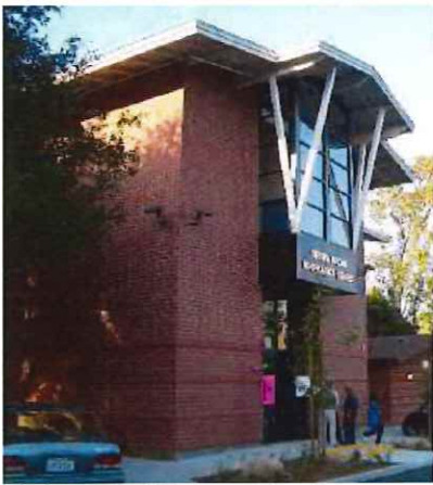
Main entry from parking lot.
