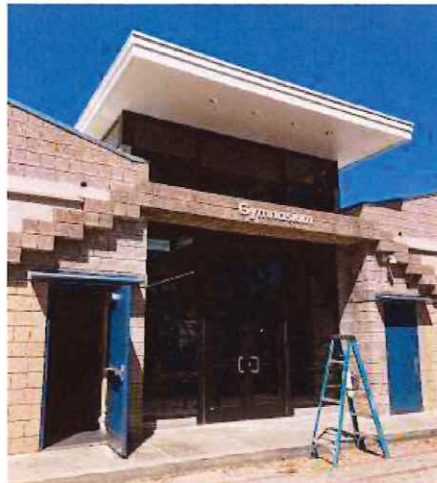
Completed Entry to Lobby of Boxing & Wt. Rm.
