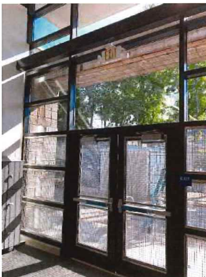
Completed Curtain-wall at New Entry Lobby
