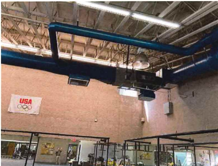
Completed new HVAC system at Boxing Gym and Wt. Rm.
