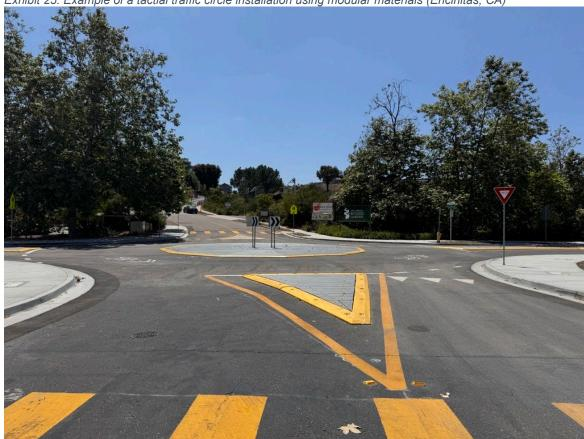
Exhibit 25. Example of a tactial traffic circle installation using modular materials (Encinitas, CA)
