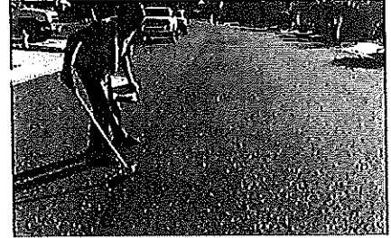
Figure 6: GMU Staff Engineer performing a PCI survey.
