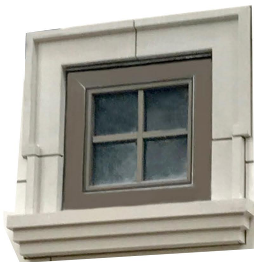
2 PRE-CAST CONCRETE MOLDINGS - MEDIUM GRAY
