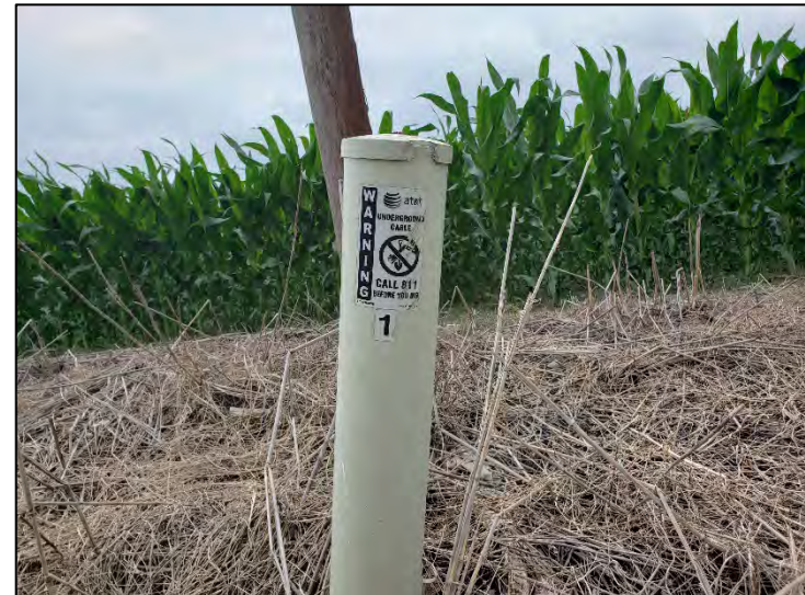
PHOTO 6 Evidence of buried cable line observed along the northern Property boundary
