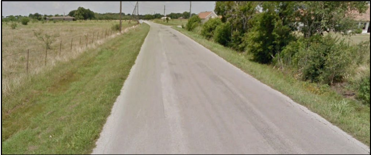
Figure 6 – Lower Seguin Road Facing West
