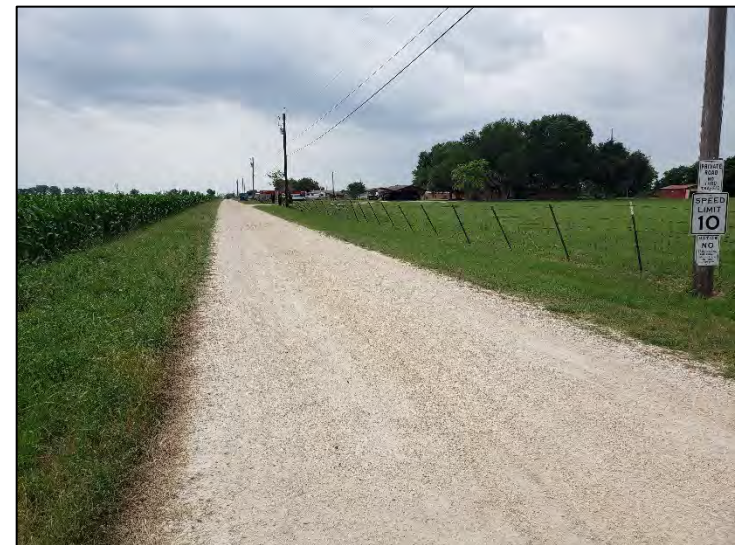
PHOTO 8 Overhead powerlines and access road located along the western Property boundary
