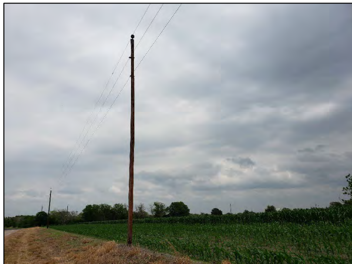
PHOTO 7 Overhead powerlines located along the northern Property boundary
