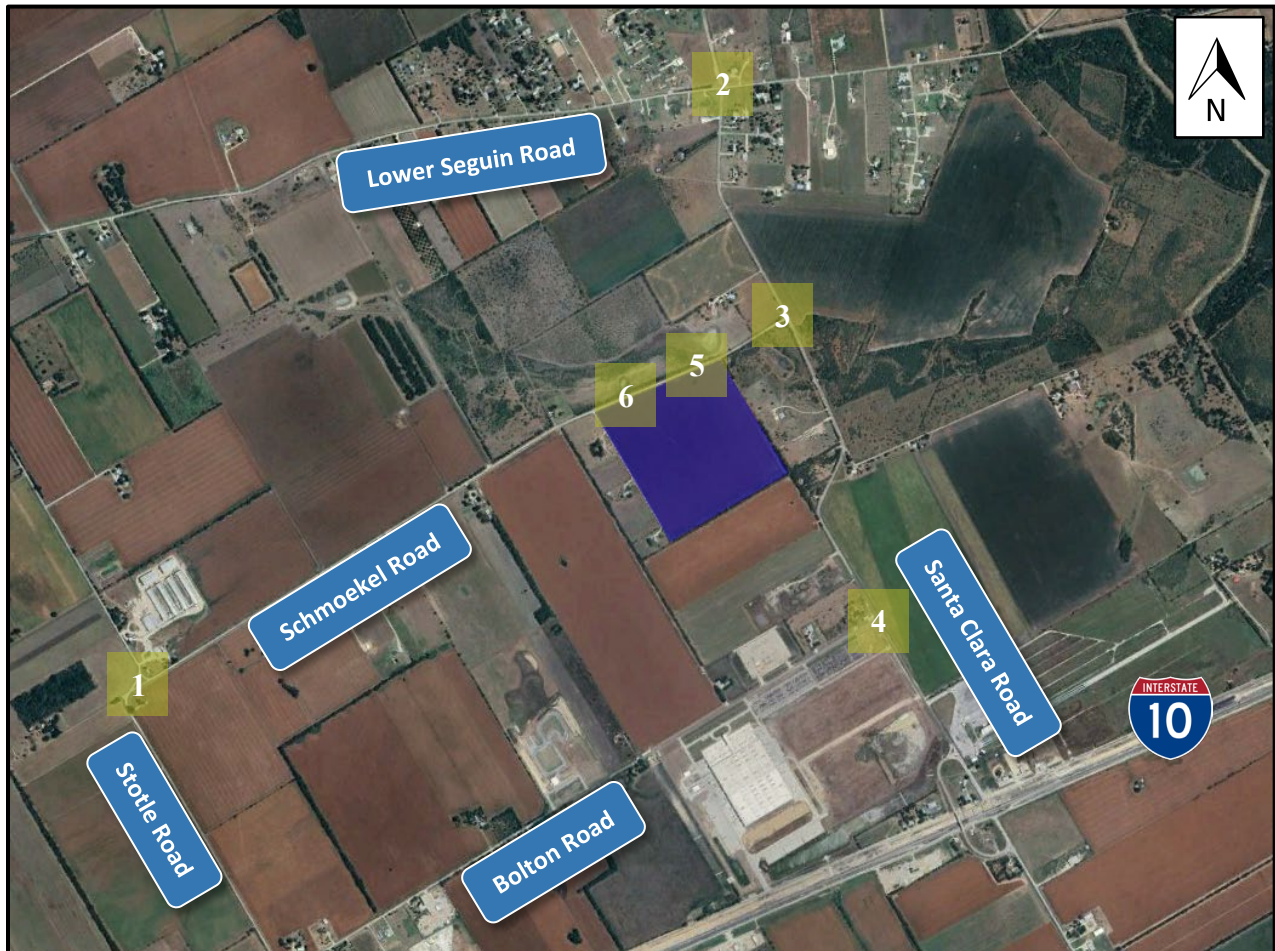
Figure 9 – Aerial with Intersections to be Analyzed
