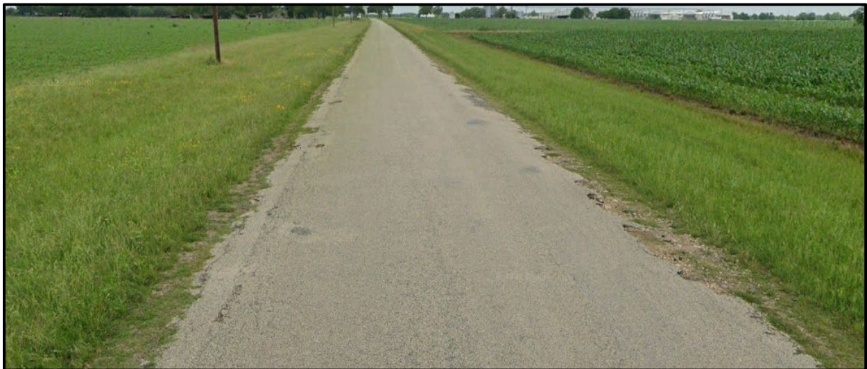
Figure 7 – Stotle Road Facing North
