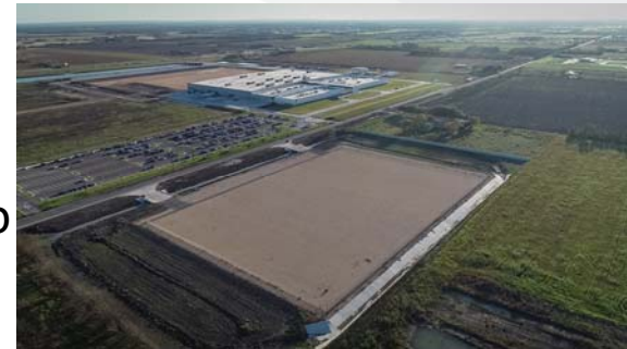
Santa Clara Substation Pad
