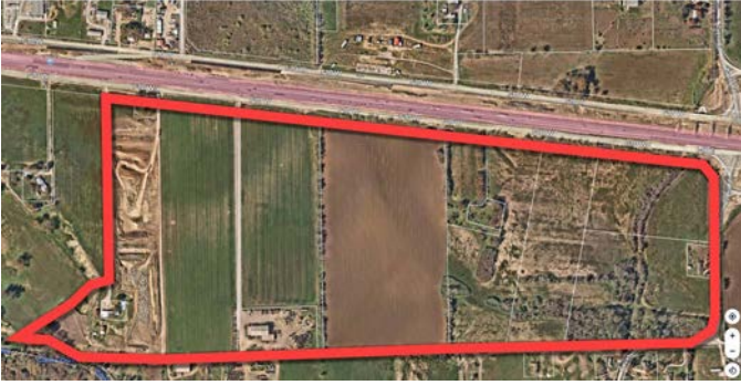
Figure 4.19 | Catalyst Site #1 -Existing Area
