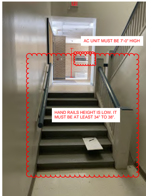
Figure 9: Stair handrails & AC unit not ADA complaint
