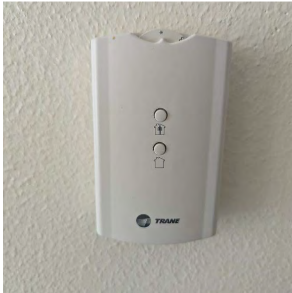
Figure 9. Second floor standalone control thermostat
