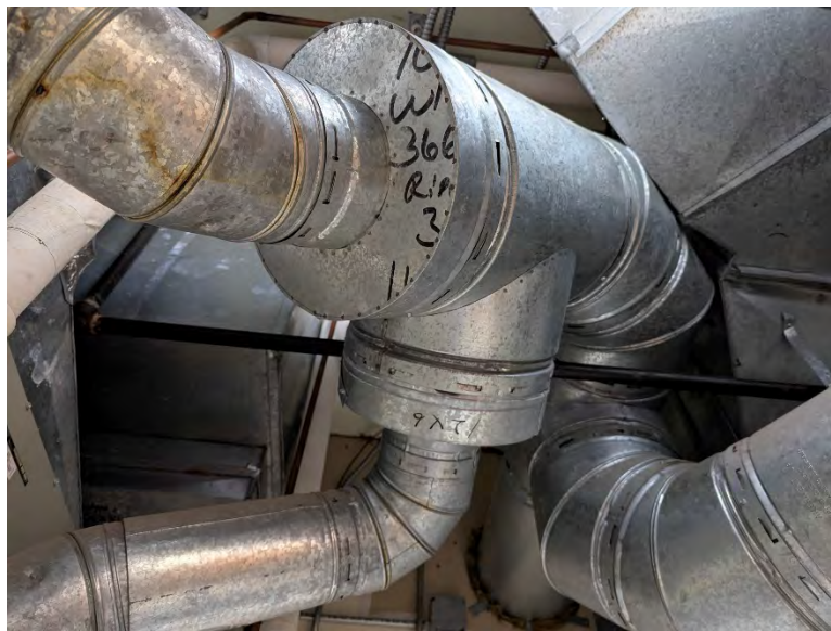
Figure 8. Various ducts tied to vertical air handlers
