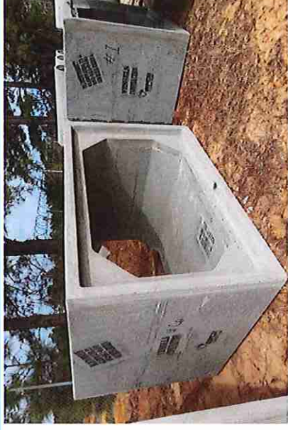
Figure 2: Proposed 8'X3' Culvert on Tolle Rd
