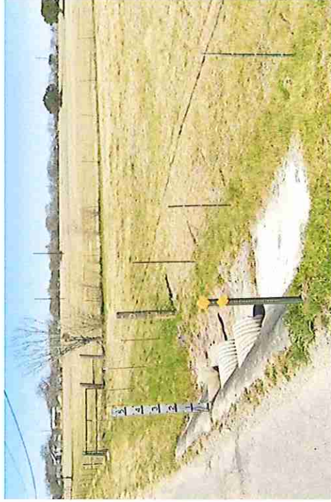
Figure 1: Existing 15" CMP on Tolle Rd
