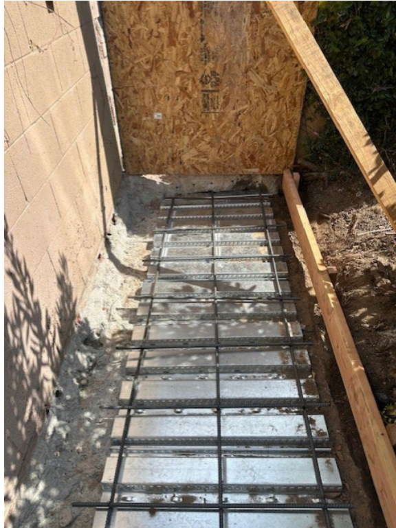
Reinforcement for culvert cover
