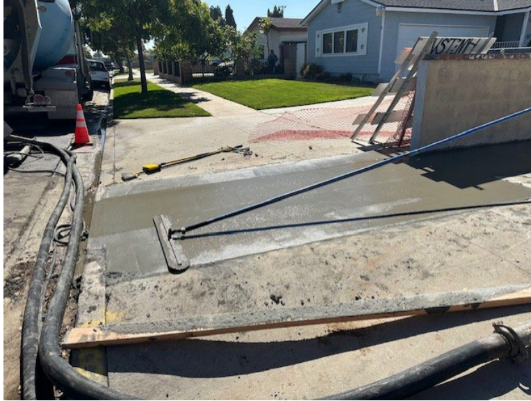
Pouring culvert cover
