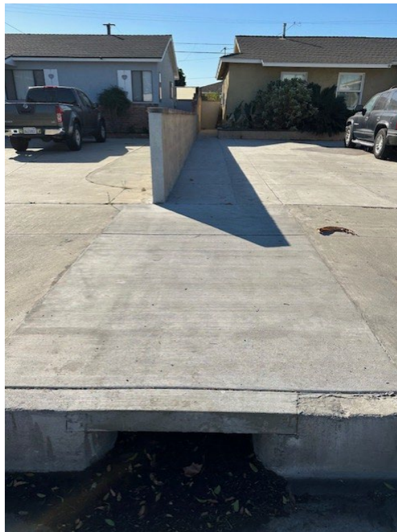
Reconstructed Culvert
