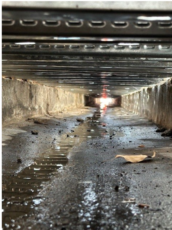
Clear passage of culvert
