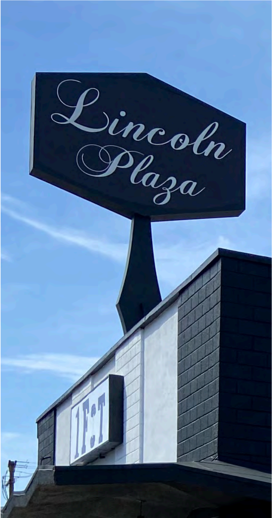
EXISTING CONDITIONS - ROOF SIGN TO REMAIN
