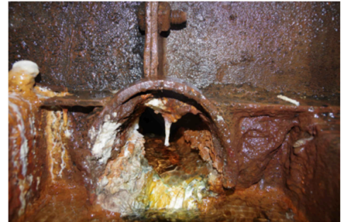
SOUTH TOE DRAIN BEFORE CLEANOUT
