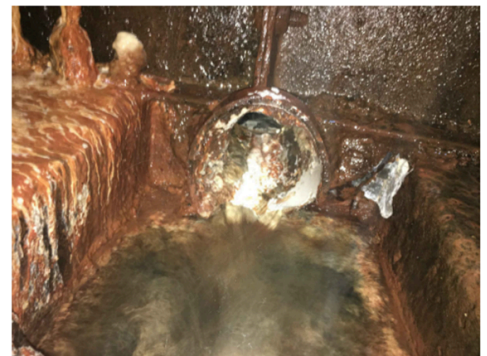
SOUTH TOE DRAIN AFTER CLEANOUT
