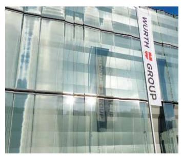
The façade of the WÜRTH Building in Switzerland is mostly glass, laminated with a fabric that is black on the inside but aluminium-coated outside. The inner surface delivers good visibility, and the fabric provides shade and interesting visual effects outside. Preliminary studies by the Swiss Ornithological Institute suggest that the materials used in this building may also deter bird collisions. Photo by Hans Schmid
