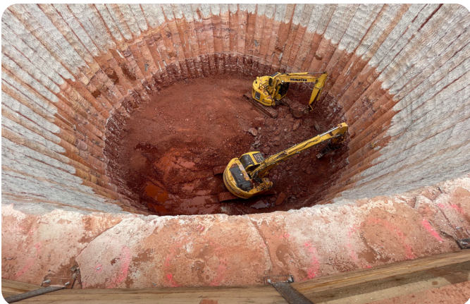
Shaft excavation at Arcadia Lake
