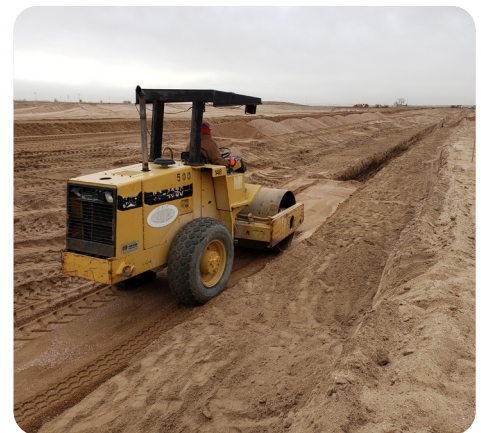
Installation of Chimney Drain inside a dam embankment
