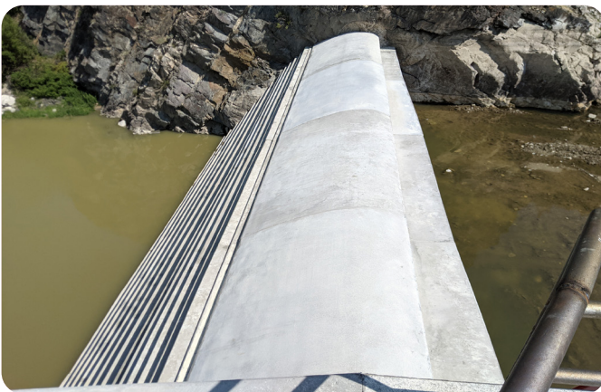
Concrete Ogee Weir at Tunnel Dam Reservoir in Wheatland, WY
