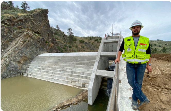
Construction oversight of ogee weir and outlet works construction at Tunnel Dam near Wheatland, WY
