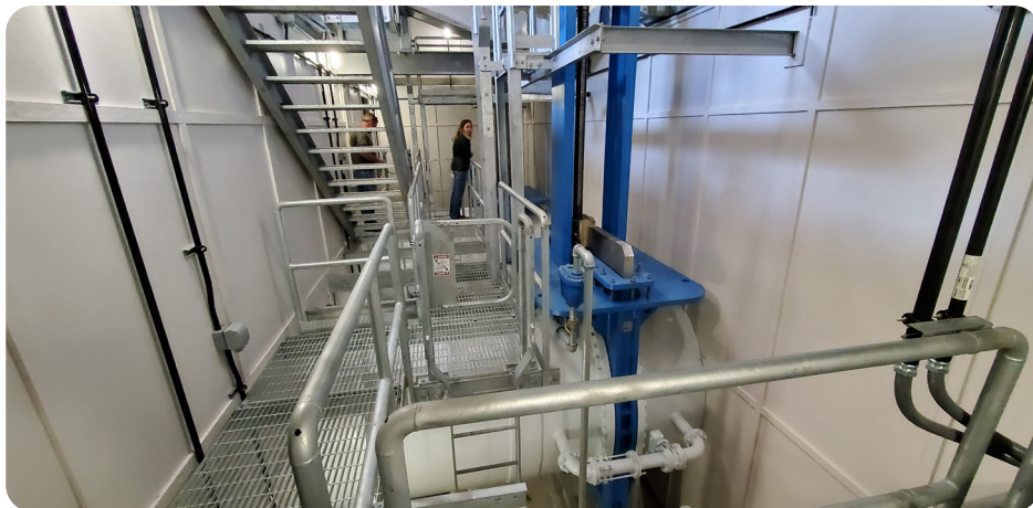
Reservoir control gates at Rio Grande Reservoir Valve House
