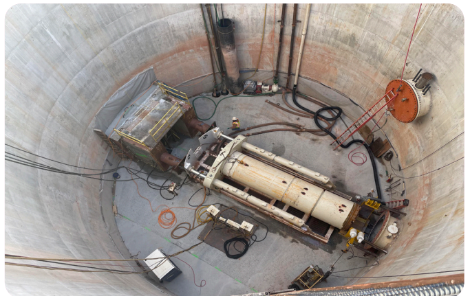
MTBM in Shaft at Arcadia Lake
