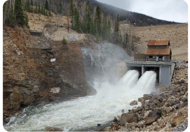
Outlet work valve house at the Rio Grande Reservoir
