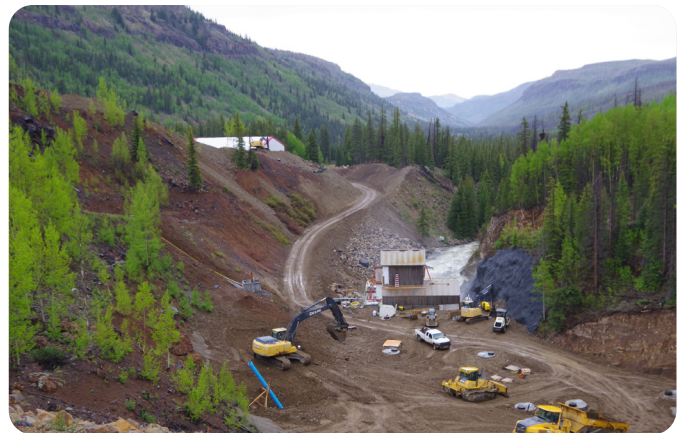
Engineered Fill and drainage material being placed along downstream toe of Rio Grande Reservoir
