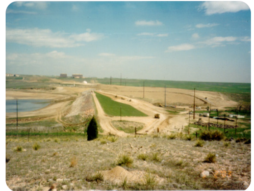
Great Western Dam Toe Berm During Construction in 2003
