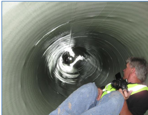
Figure 20: UV CIPP Lining of CMP Storm
