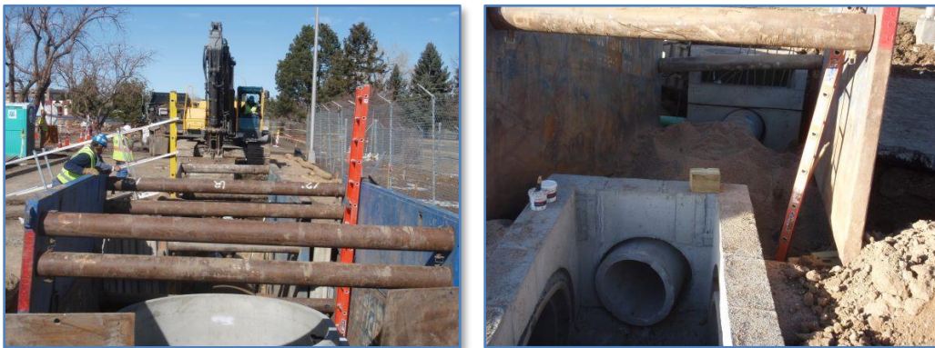
Figure 17 + 18: Storm Sewer - New Installations
