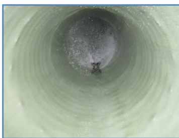
Figure 27: UV Cure CIPP/Pressure and Gravity
