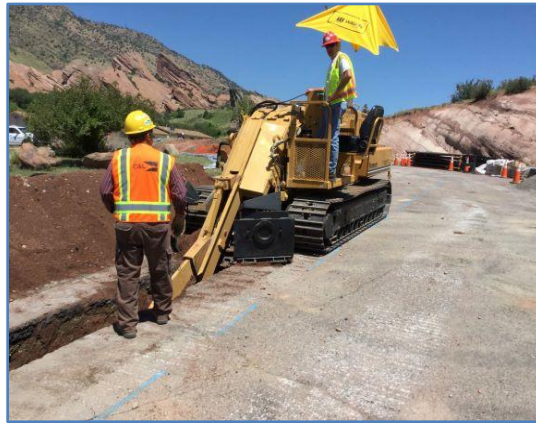
Figure 3: Water Line Install with Trencher
