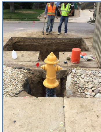
Figure 9: Fire Hydrant Replacement
