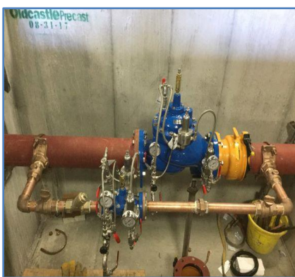
Figure 8: PRV Installation
