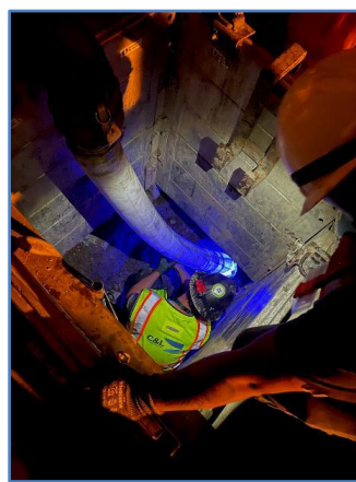
Figure 26: LED Lateral Lining
