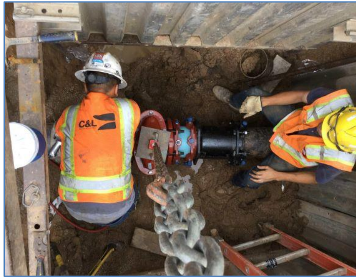
Figure 7: Valve Repairs/Replacements
