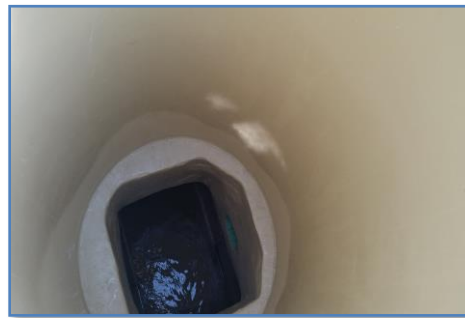
Figure 24: Manhole Rehabilitation
