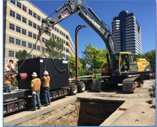
Figure 5: Butterfly Valve Vault Install
