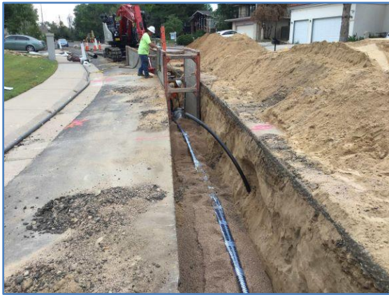
Figure 2: Open Cut Water Line R & R.
