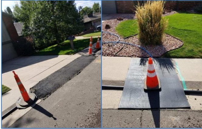
Figure 4: Temporary Water Example
