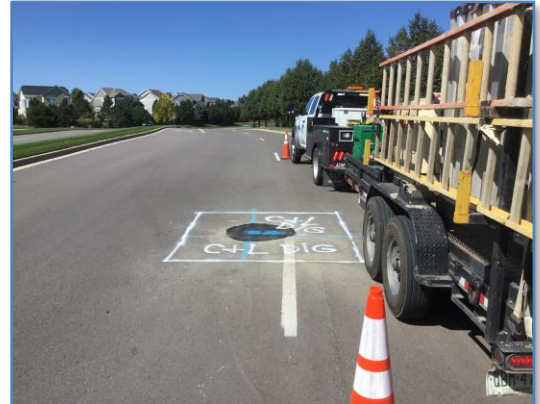
Figure 29: Water Break Layout and Crew Setup
