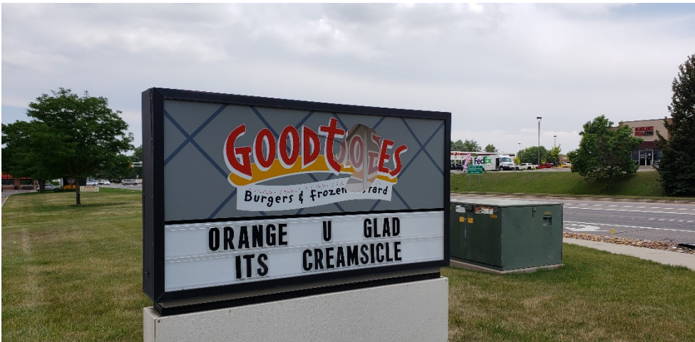
This damaged sign was located in the southern portion of the Study Area
