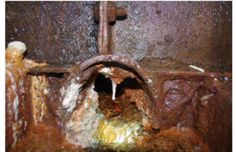
SOUTH TOE DRAIN BEFORE CLEANOUT
