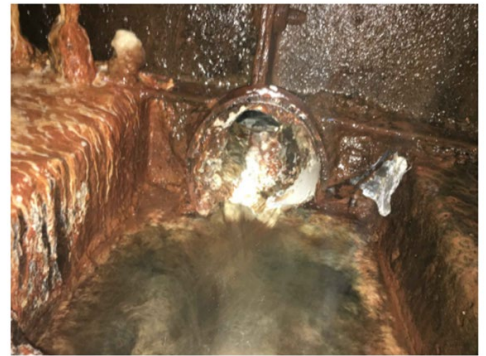
SOUTH TOE DRAIN AFTER CLEANOUT
