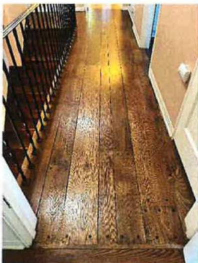
29. Interior hardwood floors A
