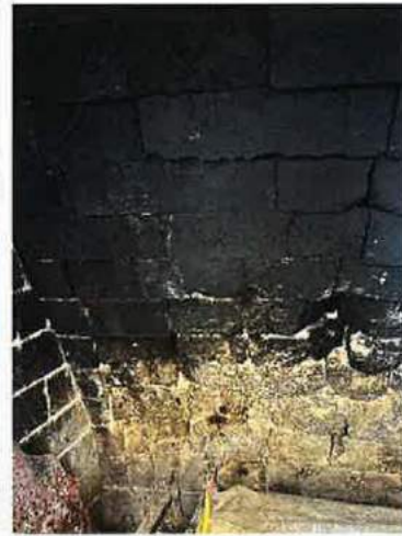
20. Interior fireplace C
