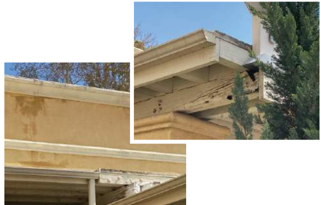
IMAGES | BUILDING MAINTENANCE & REPAIRS
