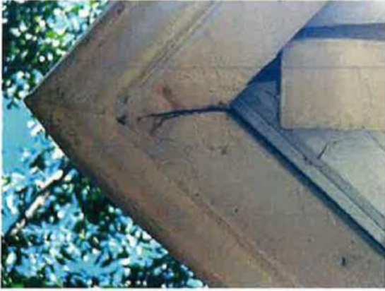
6. Gutter example A
