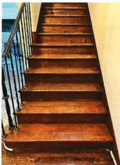
30. Interior hardwood floors B
