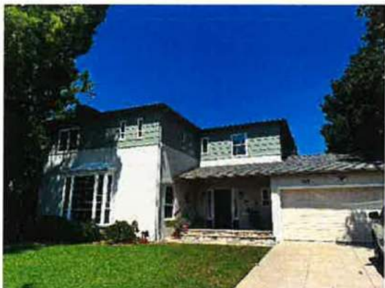
1. Exterior east view
