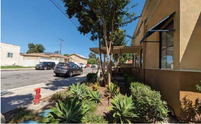
IMAGE | SENIOR CENTER - NORTH LOADING RAMP
