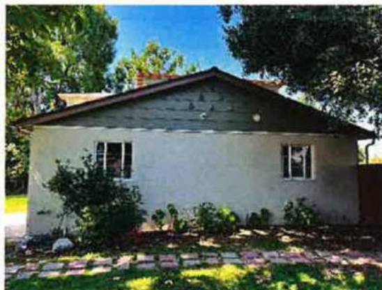
2. Exterior north view
