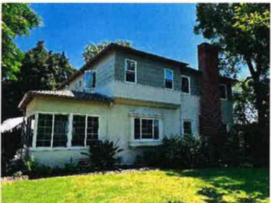
3. Exterior south view
