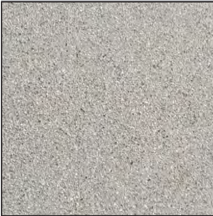
CAST IN PLACE INTEGRAL COLOR CONCRETE PAVING AT LEVEL 1 (DAVIS COLOR 'PEBBLE' WITH LIGHT ACID ETCH RETARDANT)
