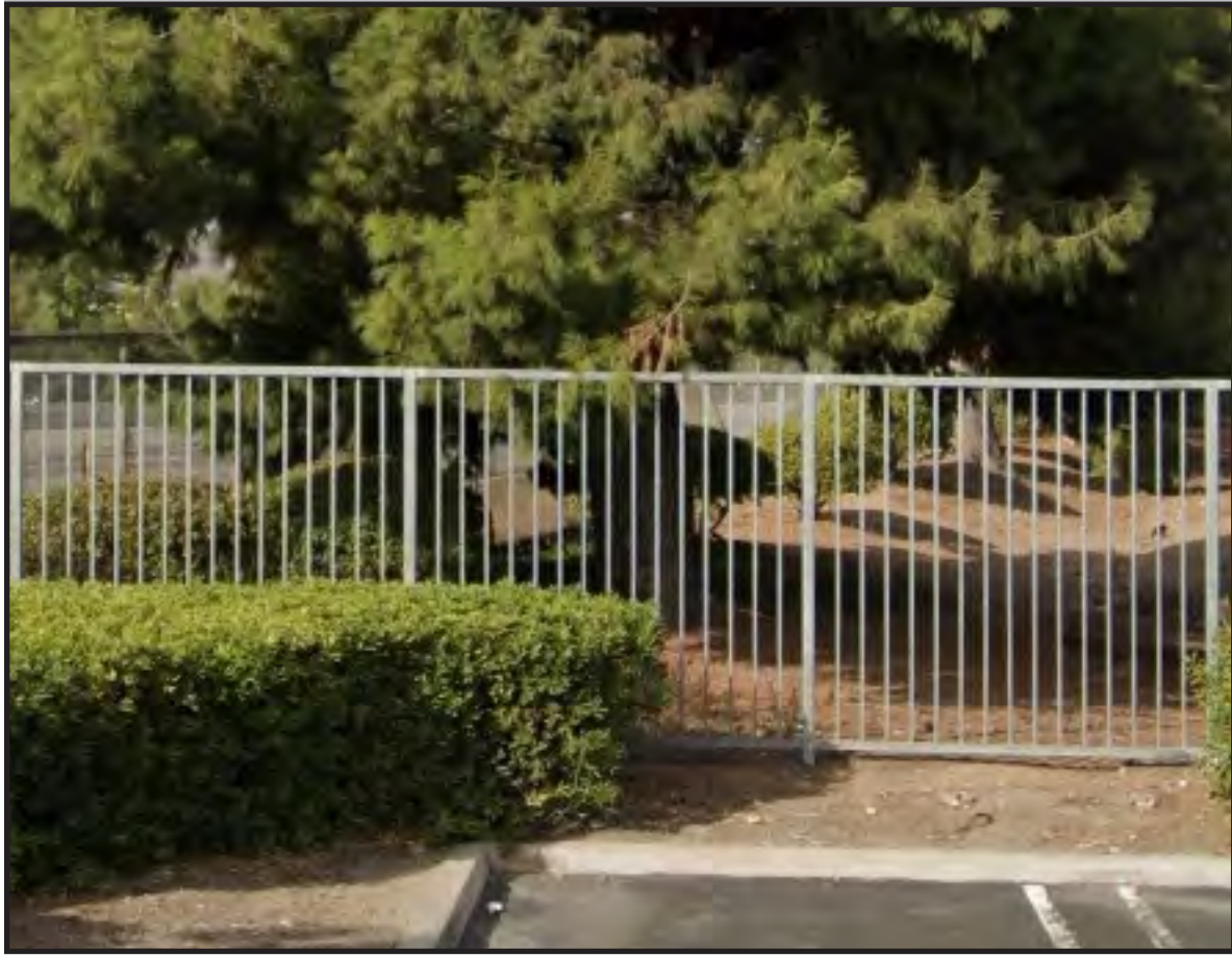
EXISTING WHITE TUBE STEEL FENCE
