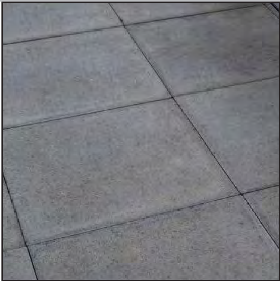
24X24 PRECAST CONCRETE PAVERS AT RESTAURANT
