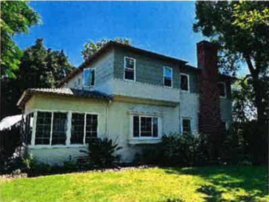
3. Exterior south view
