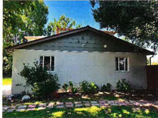
2. Exterior north view
