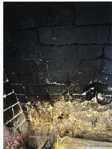
20. Interior fireplace C
