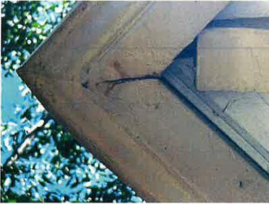
6. Gutter example A
