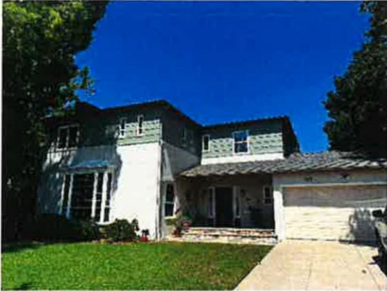
1. Exterior east view
