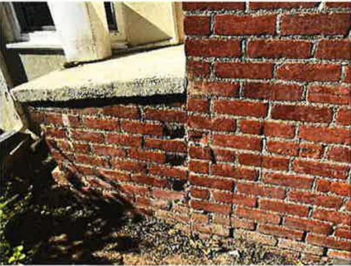
14. Fireplace exterior A
