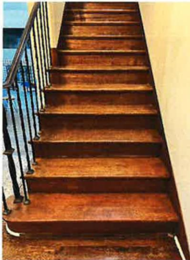
30. Interior hardwood floors B
