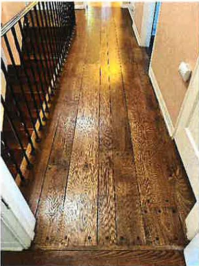
29. Interior hardwood floors A
