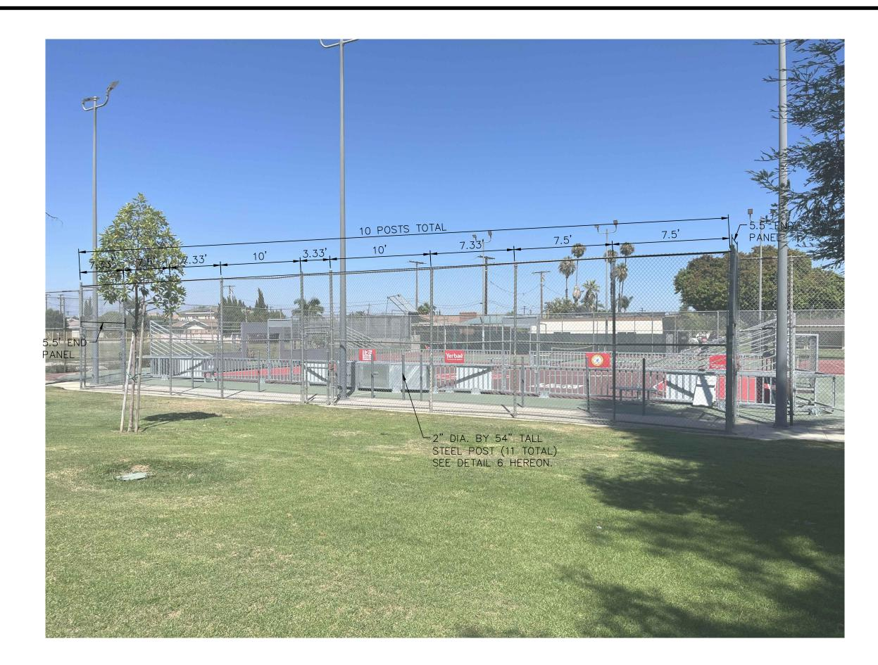
4 EXISTING 12' HIGH CHAIN LINK FENCE DETAIL C-3 SCALE: NTS
