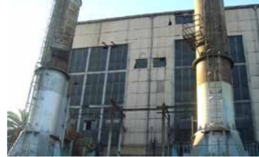
Buhar Santrali / Steam Power Plant (Uğursal, 2011)
