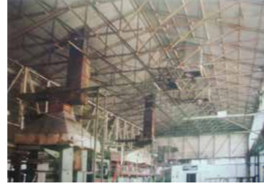
Basma İşletmesi İç Mekan / Interior of The Textile Operations Building (Şimşek, 2006)
