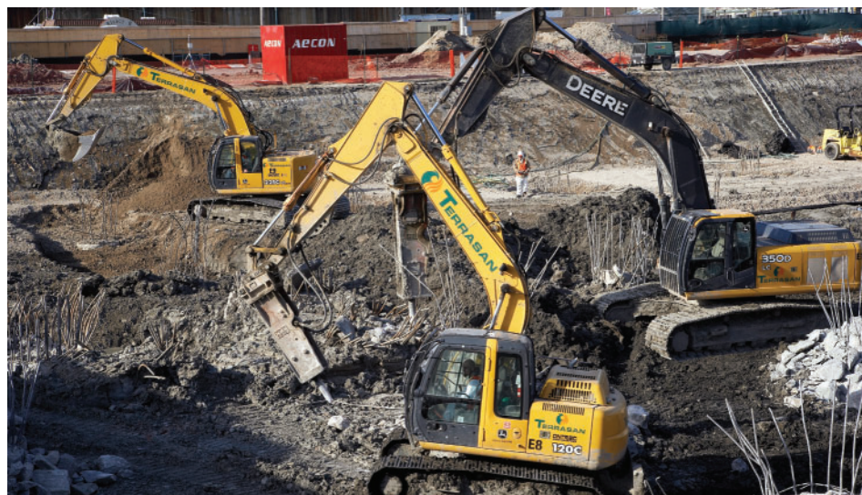
Figure 1 The process of excavating and treating large tracts of contaminated land is very costly and disruptive.
