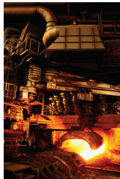
Figure 5 An exhaust hood (near the top of this photo) prevents any vapours or dust from leaving the process.
