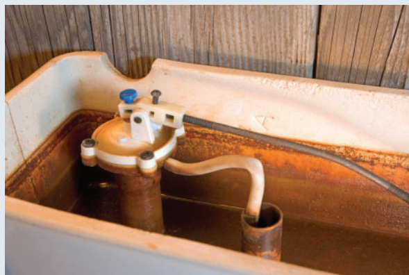
Figure 6 The brown stain inside this toilet tank is caused by a high concentration of iron(III) ions in the water supply.
