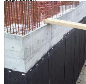
Figure:5 Second coat application
