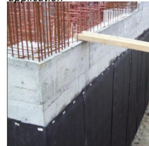
Figure: 4 Second coat application
