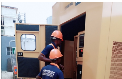
500 KVGENERATOR AND CHANGEVER PANEL INSTALLATION AND COMMISSIONING
