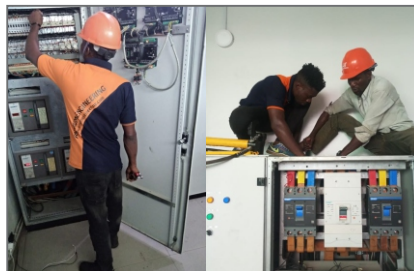
CONSTRUCTION AND INSTALLATION OF 1600A & 2500A SYNC/ATS AND ATS/D.B PANELS
