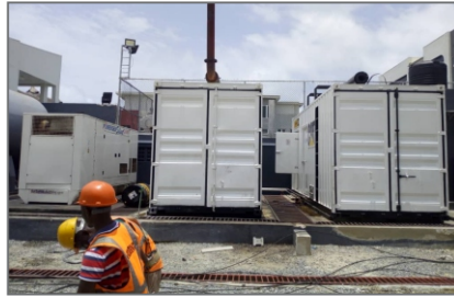
2.2 MVA BACKUP POWER GENERATORS (2 X 800KVA + 1 X 600 KVA) INSTALLATION AND MAINTENANCE
