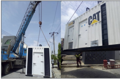
2.2 MVA BACKUP POWER GENERATORS (2 X 800KVA + 1 X 600 KVA) INSTALLATION AND MAINTENANCE
