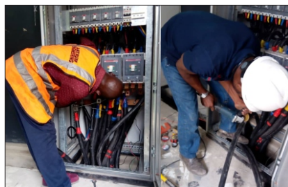
1600A DISTRIBUTION PANEL CONSTRUCTION AND INSTALLATION
