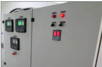
CONSTRUCTION AND INSTALLATION OF 1600A & 2500A SYNC/ATS AND ATS/D.B PANELS
